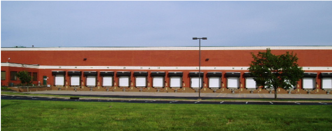
Figure 3 (Photo 1): Warehouse & Distribution Center, Monroe Township, NJ
